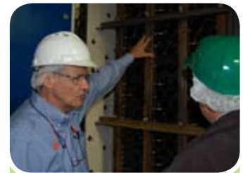
General Mills' John Hellweg spearheaded the biomass burner project.
